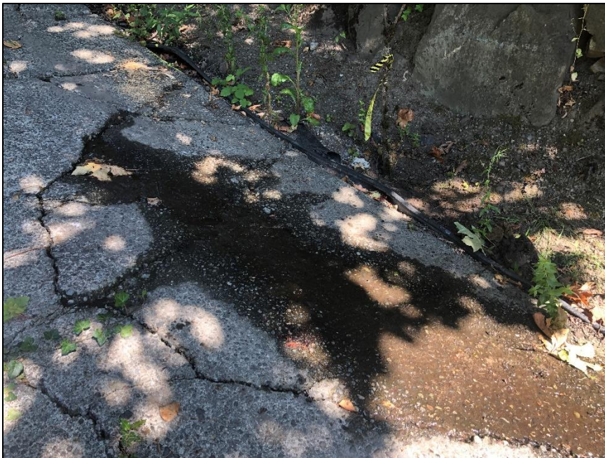
Photo 6. Surface seeps coming out of driveway adjacent to Wetland A (photo taken 7/23/21).
